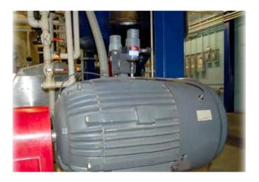
In the Lubrication Engineers manufacturing facility, we use a Xport Star Vario Single-Point Lubricator filled
